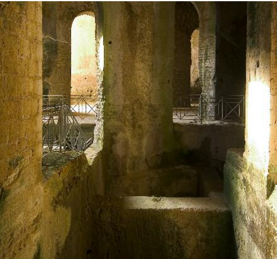
Bacoli - Cento Camerelle Bacoli - Cento Camerelle cistern
